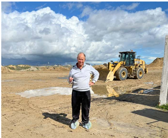
Mud alongside the storage sheds. Note the approved footwear for container access. The clouds were spectacular.
